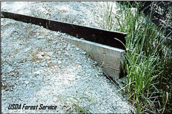
Water deflectors are installed so that 3 inches of rubber belting extends above the surface of the road.
