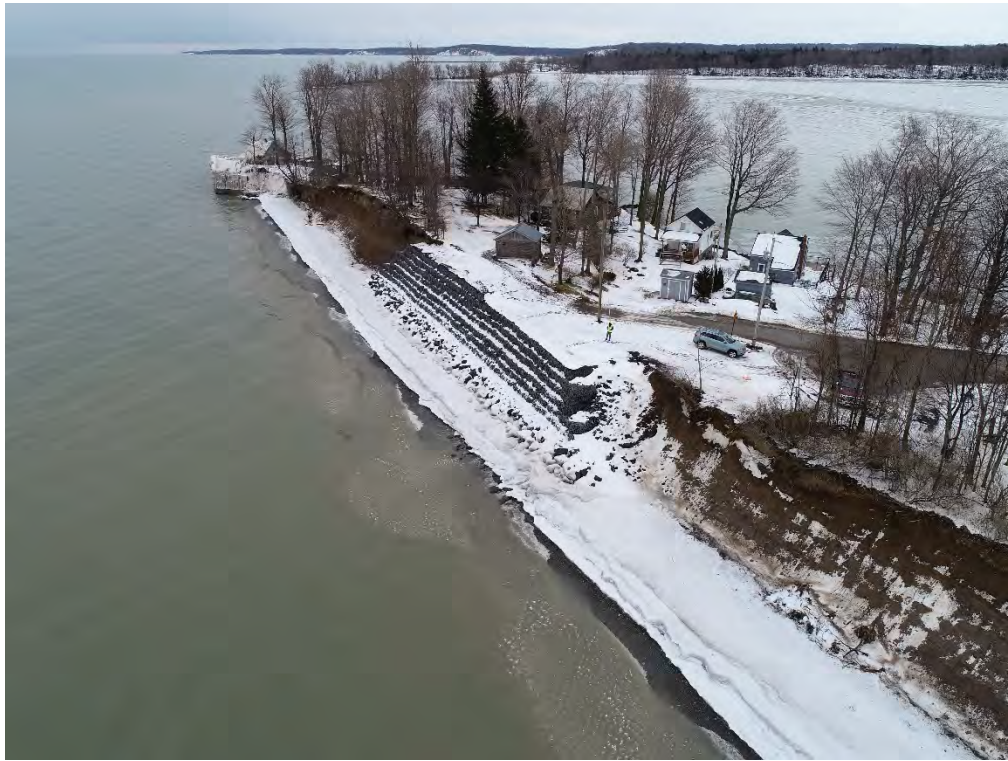
Figure 4-2 Recently constructed gabion wall
