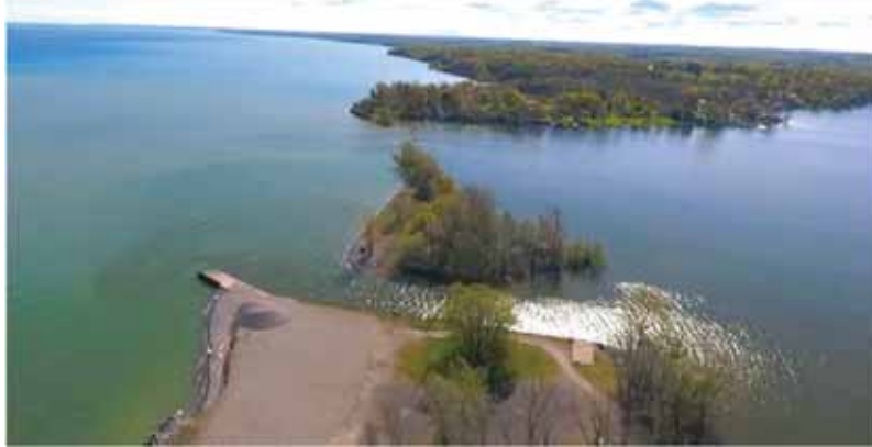
East barrier bar breach wide open because of high water level
