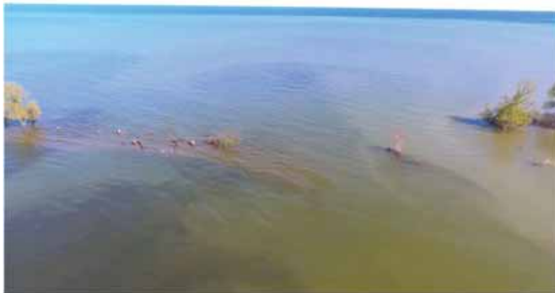
Part of the east barrier bar (repair of 2016, west of the breach) inundated because of high water level
