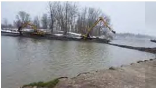
Dredging on Apr. 6, 2016; looking south
