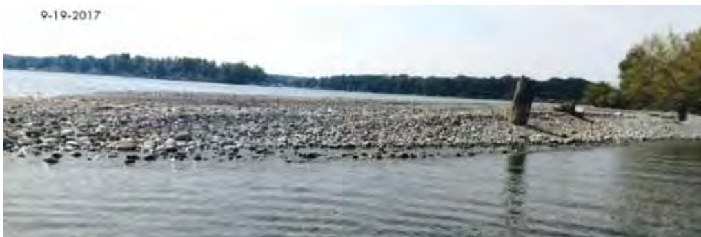
Location of the 2016-repair as of Sep. 19, 2017 9 (~WL 246.2)
