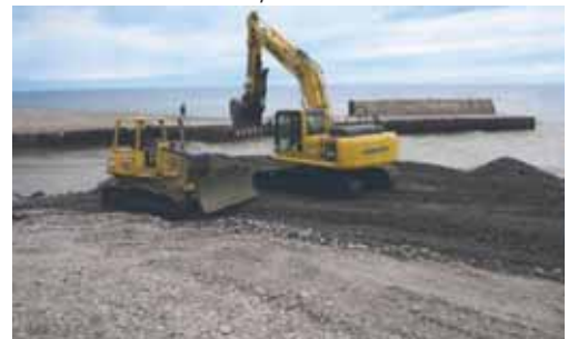
Access to the east side of the channel is critical for proper dredging and placement of materials on east bar
