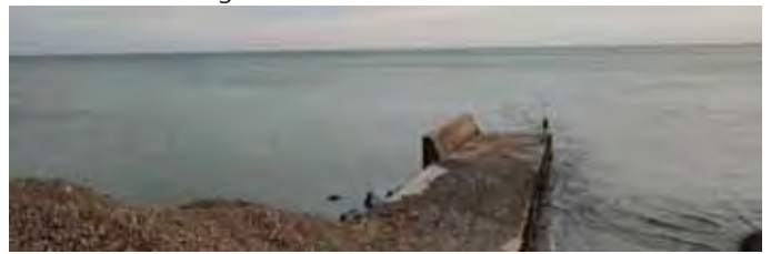
(a) Pile of gravel on the pier next to concrete wall from longshore sediment transport (LST); looking northeast (Drone view, Mar. 27, 2018; Photo credit: David Aldrich, PBIA)
