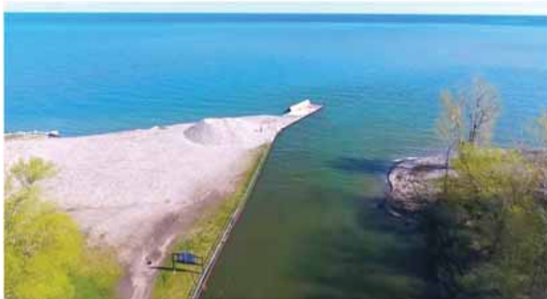
Pier, spoil area (dredged materials), and head of the east barrier bar
