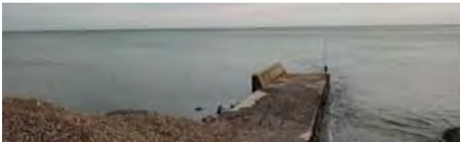
Part of dredged materials (spoil #1) near the pier; looking north
