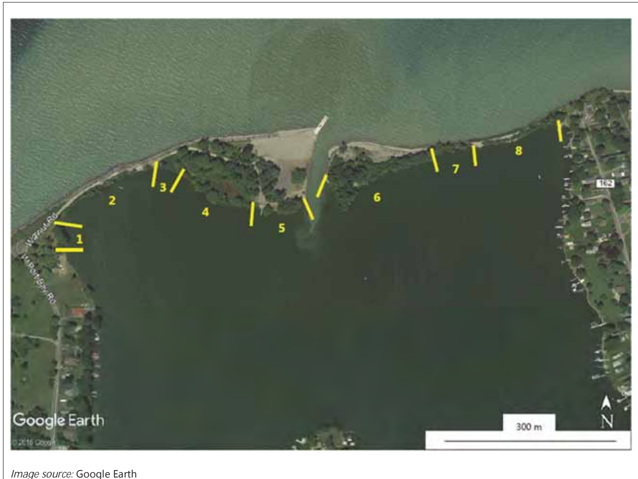
Figure 2.3-2 Littoral Zone Habitat Segments Identified along the Bay Side of the Port Bay Barrier Bar during the Littoral Zone Characterization, Jun. 22, 2018
