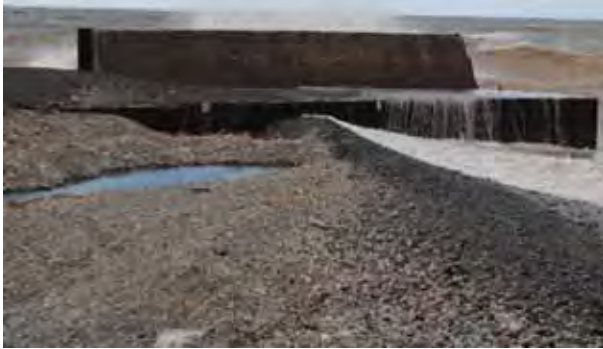
Filled-in navigation channel outlet; looking northwest. Note gravel on the pier.
