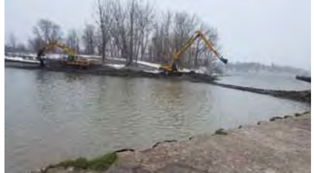
Dredging on April 6, 2016; looking south. Note gravel bar across the entire outlet.
