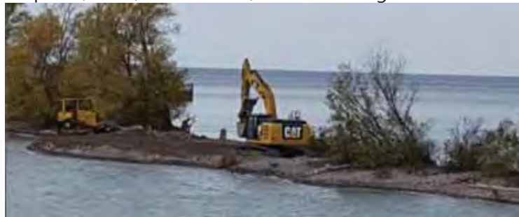
Repair completed in Nov. 2016 (~WL 244.4 IGLD85)
