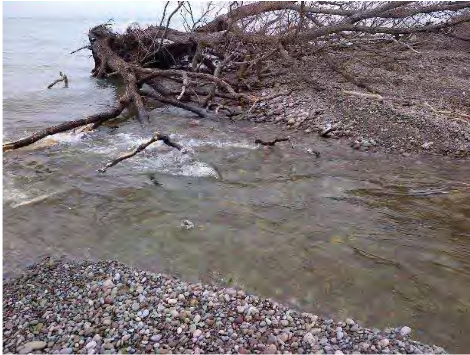
Figure 2.1-46 Sediment Near the Breach (gap) in the East Barrier Bar, Mar. 7, 2018
