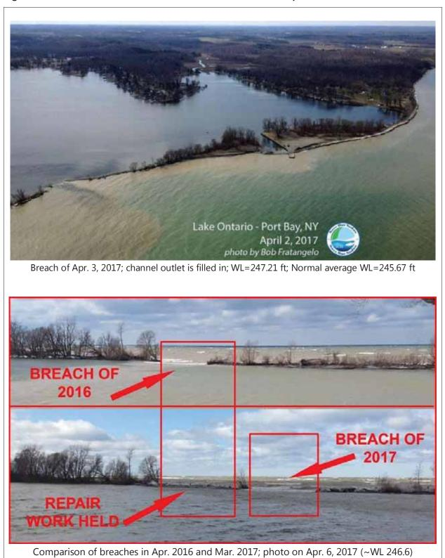
Figure 2.1-10 East Barrier Bar Breaches of 2017 and 2016 Compared
