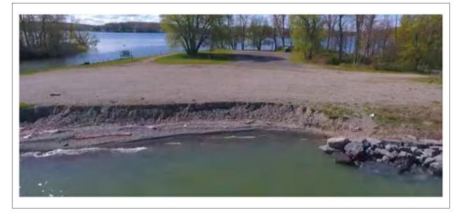
Figure 2.1-34 Wave-Induced Bank Erosion West of the Pier, May 10, 2017 (drone view)
