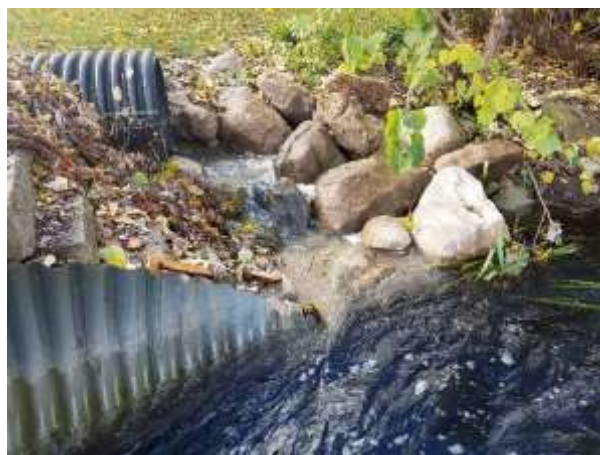
Two separate dates (Top- 6/15/17, Bottom- 10/30/17), stormwater drain discharging turbid water at RCE 9. Possible source is material stockpiles at Marion Highway Department.
