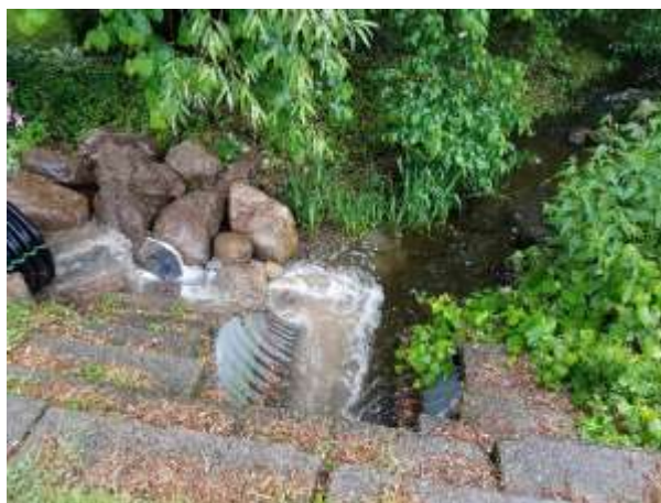
Two separate dates (Top- 6/15/17, Bottom- 10/30/17), stormwater drain discharging turbid water at RCE 9. Possible source is material stockpiles at Marion Highway Department.
