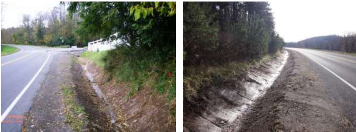
Unseeded roadside ditch observed in the Lower Ganargua Creek Watershed.
