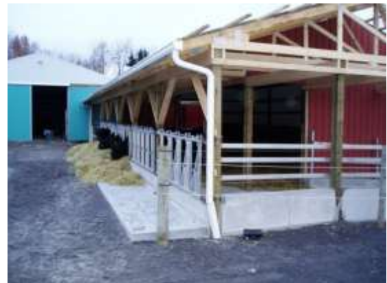
Left: Example of a barnyard management plan designed to contaminated runoff. Below: Installed barnyard management
