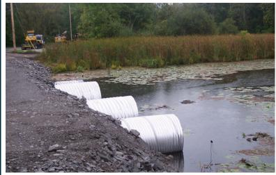
In 2024, The district completed a culvert replacement project along West Port Bay Road in the Town of Huron. Previously, a single dilapidated culvert connected the Beaver Creek wetland complex to the southwestern side of Port Bay.
