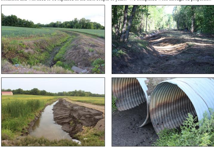
**Ki-Ham-Law Project:** This project is <sup>3</sup>/<sub>4</sub> of a mile long and located in the town of Macedon. The project was mowed and dipped. Due to the depth of the ditch, this project requires a long stick excavator to dip. The work on this project provides good drainage to a 30-acre piece of muck land.
