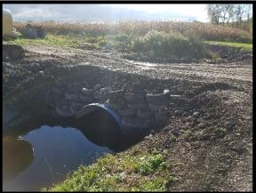
Melvin Brook: This maintenance project is in the town of Galen and is about 1.5 miles long. We mowed and removed blockages on the entire project and cleared willows along one side of the ditch that had been skipped the last couple maintenance cycles. We also ordered pipe to replace two failing culvert crossings but due to poor weather we were not able to install the pipes this fall.
