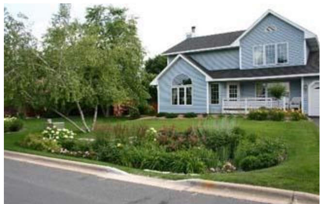
Rain garden that collects stormwater from the house and from the street. Photo from US EPA.
